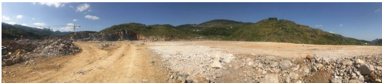
Site leveling underway - new Finlays secondary processing facility, Sinan, Guizhou, China
